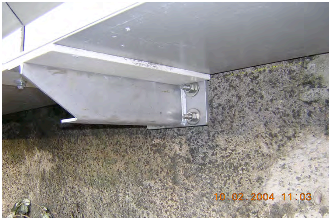
CABSYS RAIL an Betonwand
